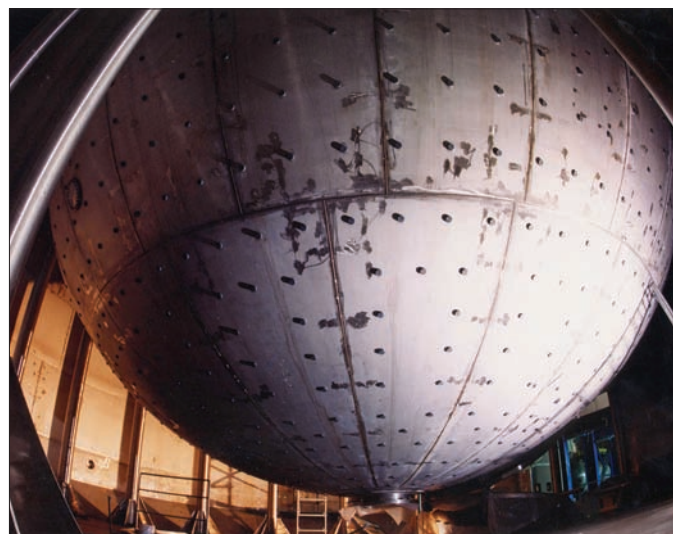
The Borexino stainless-steel sphere. It serves both as a support structure for the 2200 photomultipliers that detect the scintillation light and as a container for the inner part of the detector, which consists of a nylon balloon with 278 t of scintillator surrounded by a buffer liquid (950 t). (Courtesy INFN–Gran Sasso National Laboratories.)
