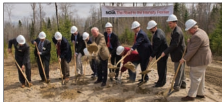
Ground-breaking gives the NOvA project an official start. (Courtesy Fermilab Visual Media Services.)
