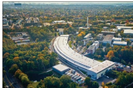
The new hall on PETRA III. (Courtesy DESY.)
